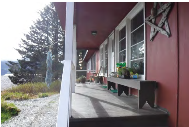
Blair House – Main residence (4)
