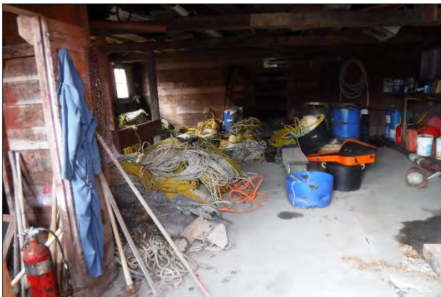
Interior Beach Locker Building
