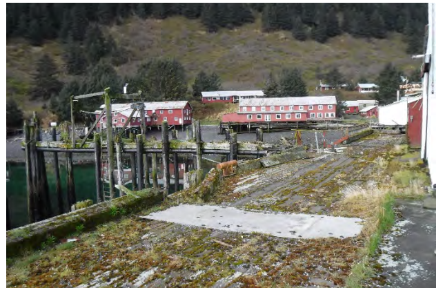
East side of main dock
