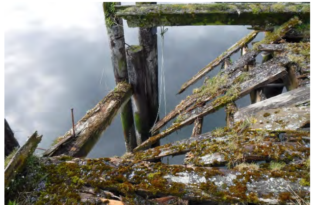
North end of the east side of dock
