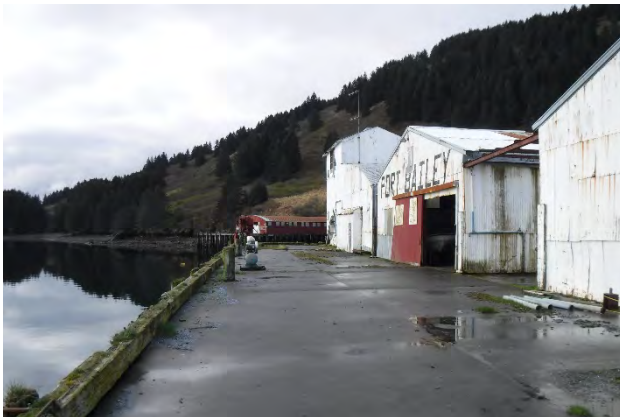
East view along Main Dock
